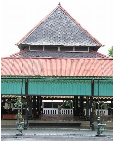
Figure 1. Sultan's palace joglo at Srimanganti Hall
